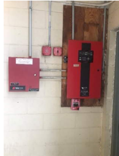
Fire Alarm System – Six Bay Vehicle Storage Garage
