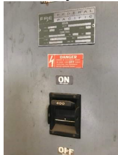
400 Amp, 240 V1, 1-Phase Main Building Disconnect – Mezzanine of Six Bay Vehicle Service Storage Garage
