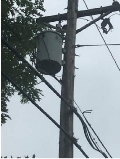
Service Transformer on Depot Road
