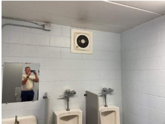
Bathroom Transfer Fan from Breakroom
