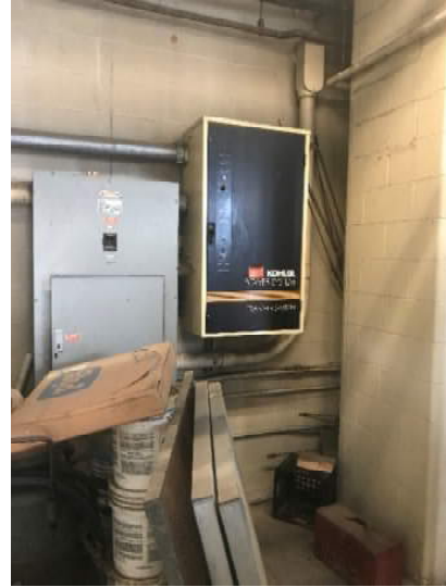
400 Amp Automatic Transfer Switch – Mezzanine of Six Bay Vehicle Storage Garage
