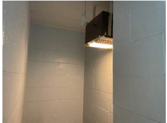
Bathroom Ceiling Exhaust Fan
