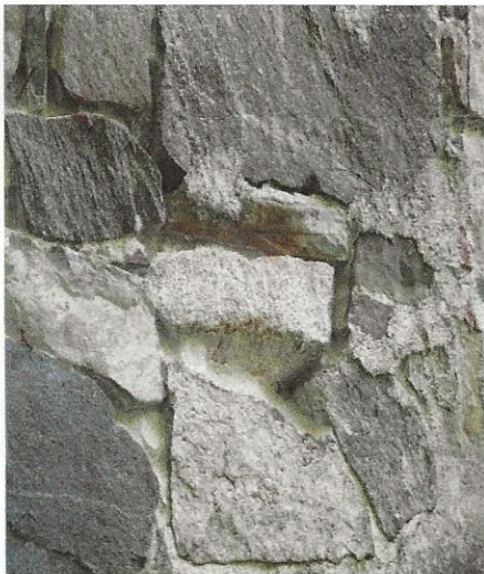
(Missing mortar)
