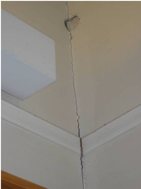
Crack in interior plaster finish
