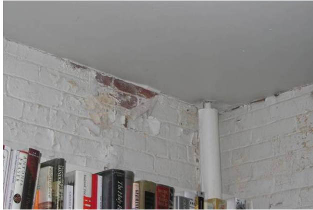
Typical Water damage to paint on basement bricks
