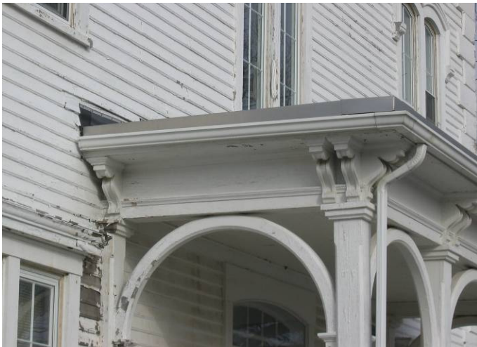
Roof repair and siding damage at front porch area
